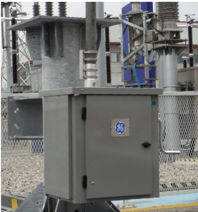
Typical installation of DWatch mechanism - external view
